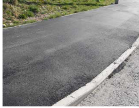
Bitmac pedestrian surfacing
