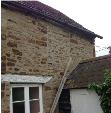
Fig.29 - Evidence of former opening and later extension
