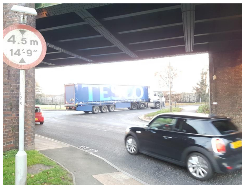
Photo 3.2.3 Example of HGV on wrong side of road turning right
