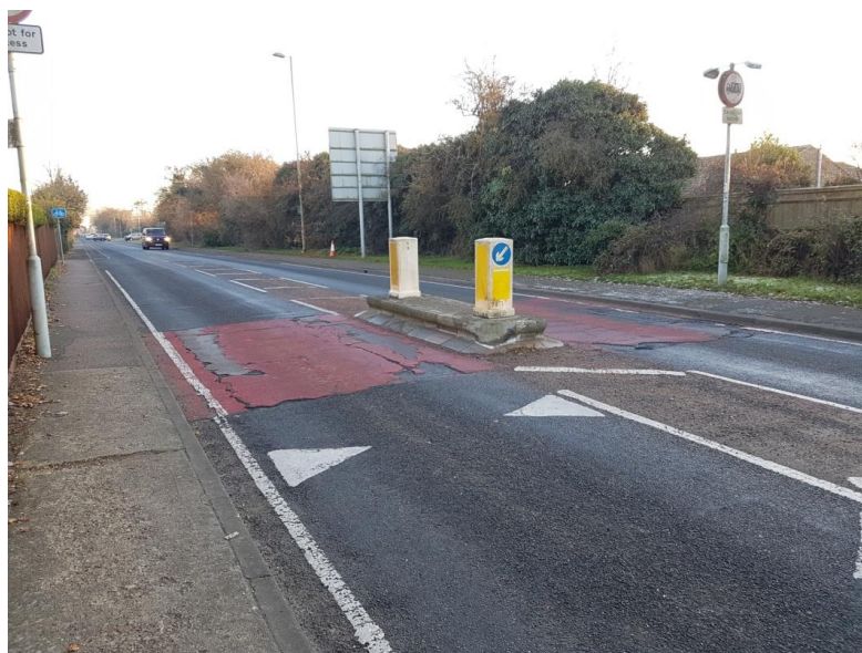
Photo 3.3.4 Existing Central Island
