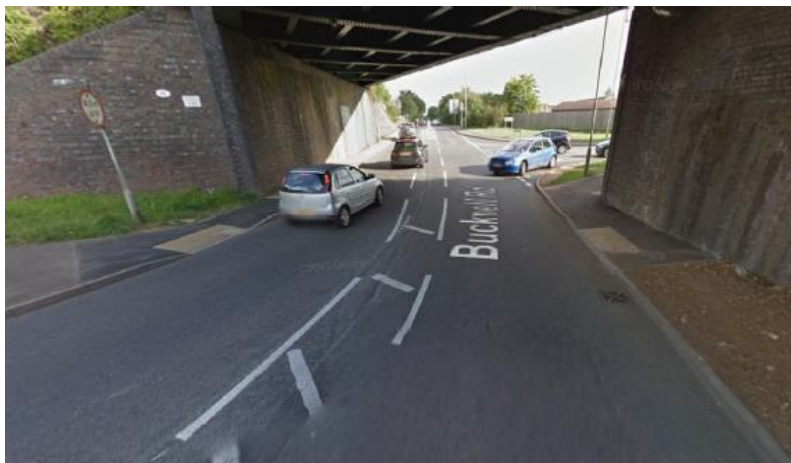
Photo 3.3.2 Dropped crossing under Railway Bridge (@googlemaps)
