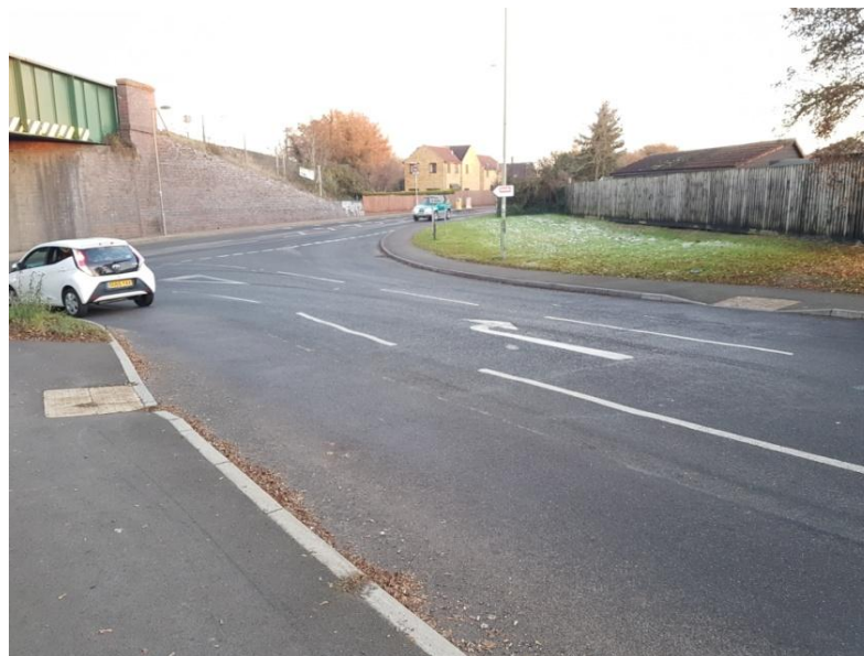
Photo 3.3.1 Location of dropped crossing on Howes Lane
