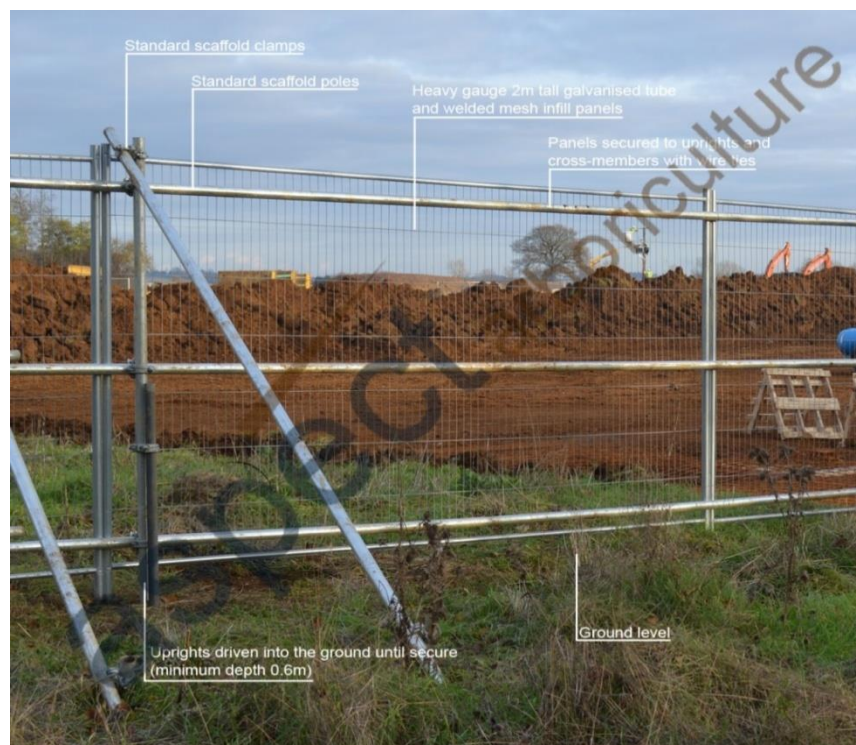
Plate.1 Default Protective Barrier Specification
