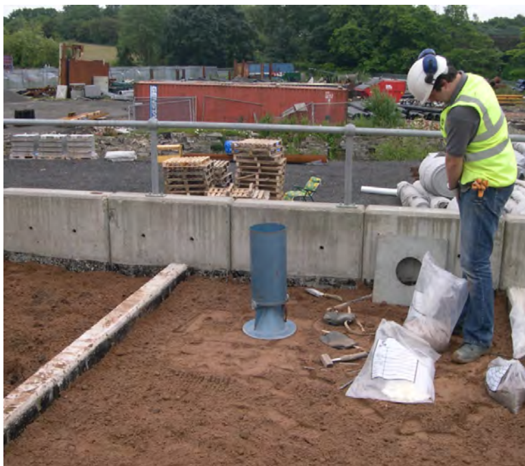
Figure 1 - In situ density test prior to construction of pavement.
