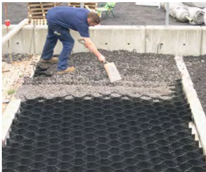
Figure 2 - CellWeb TRP® in construction.
