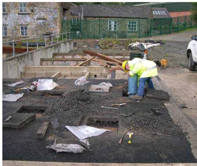
Figure 3 - In situ density tests post-trafficking.
