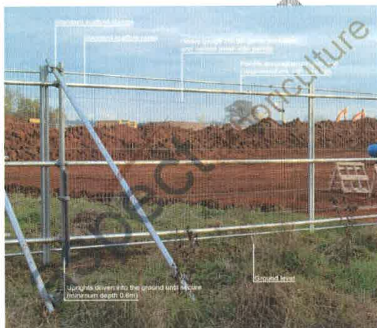
Plate.1 Default Protective Barrier Specification
