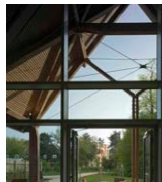
Glazed curtain wall & extended roof canopy
