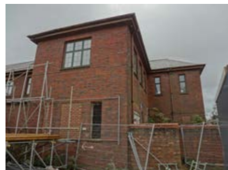
Re-instating bricked up windows
