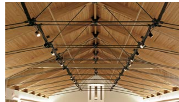
Glulam timber with slender steel bracing
