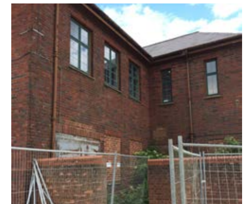
Demolition of courtyard walls
