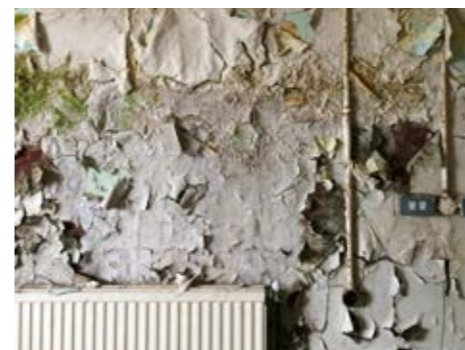
Damp brickwork
