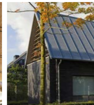
Metal standing seam roof finish
