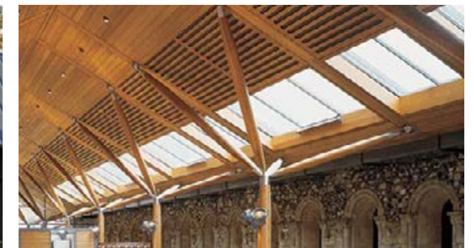
Circular columns and struts
