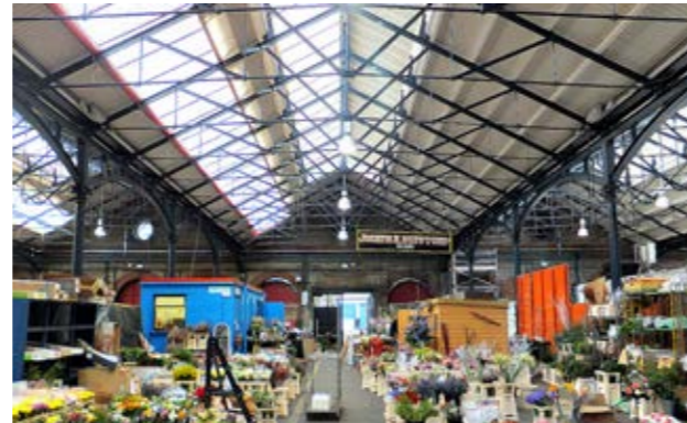
Long span trussed roof form
