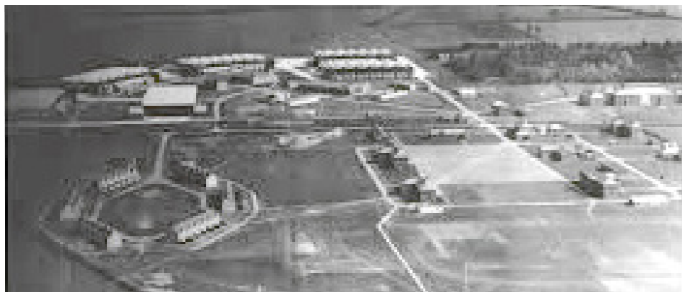
Aerial photograph of the site in 1928
