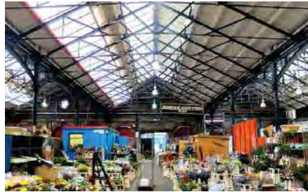
Long span trussed roof form
