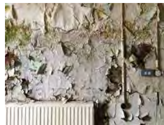
Damp brickwork
