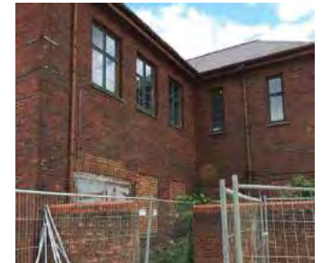
Demolition of courtyard walls
