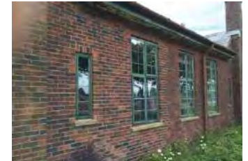
Tall windows on southern elevation
