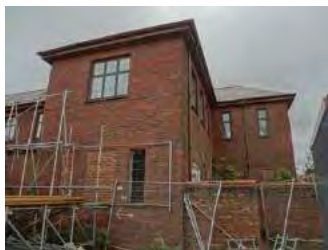
Re-instating bricked up windows
