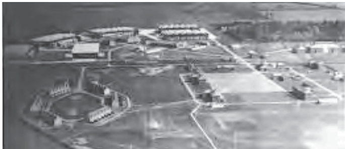
Aerial photograph of the site in 1928
