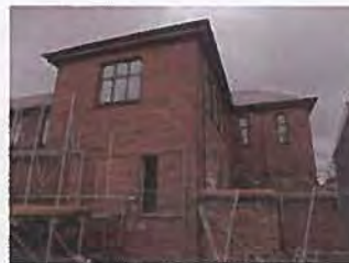
Re instating bricked up windows
