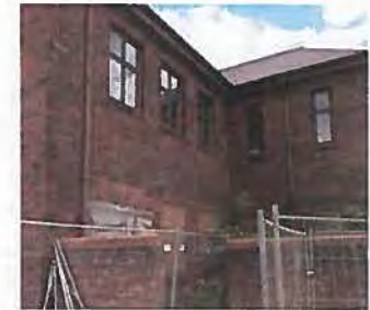
Demolition of courtyard walls
