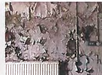
Damp brickwork
