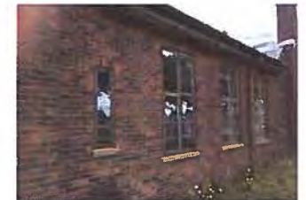
Tall windows on southern elevation
