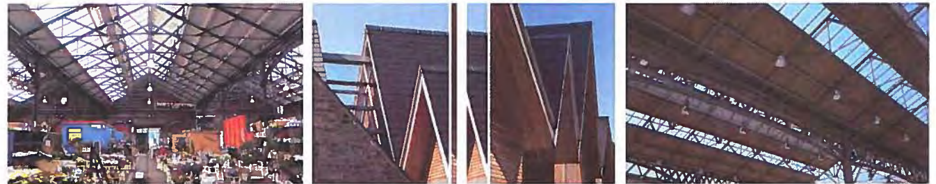
Long span trussed roof form
