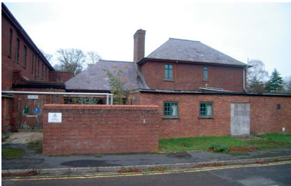
Plate 3: South side of Building 455
