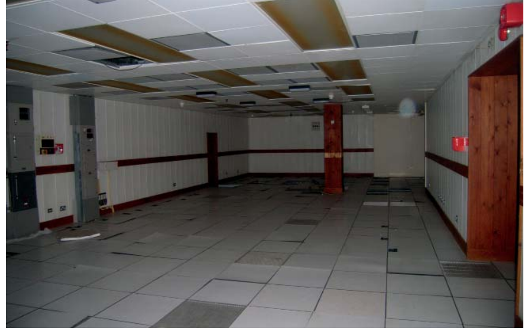
Plate 6: Ground floor room in main range of Building 455
