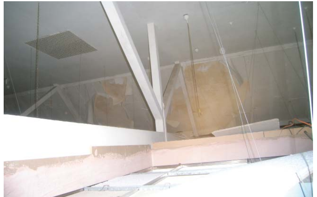
Plate 8: King post truss above later suspended ceiling in Building 455
