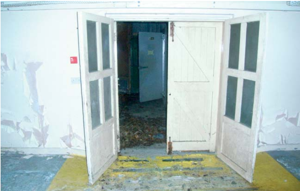
Plate 15: Doorway within Building 457
