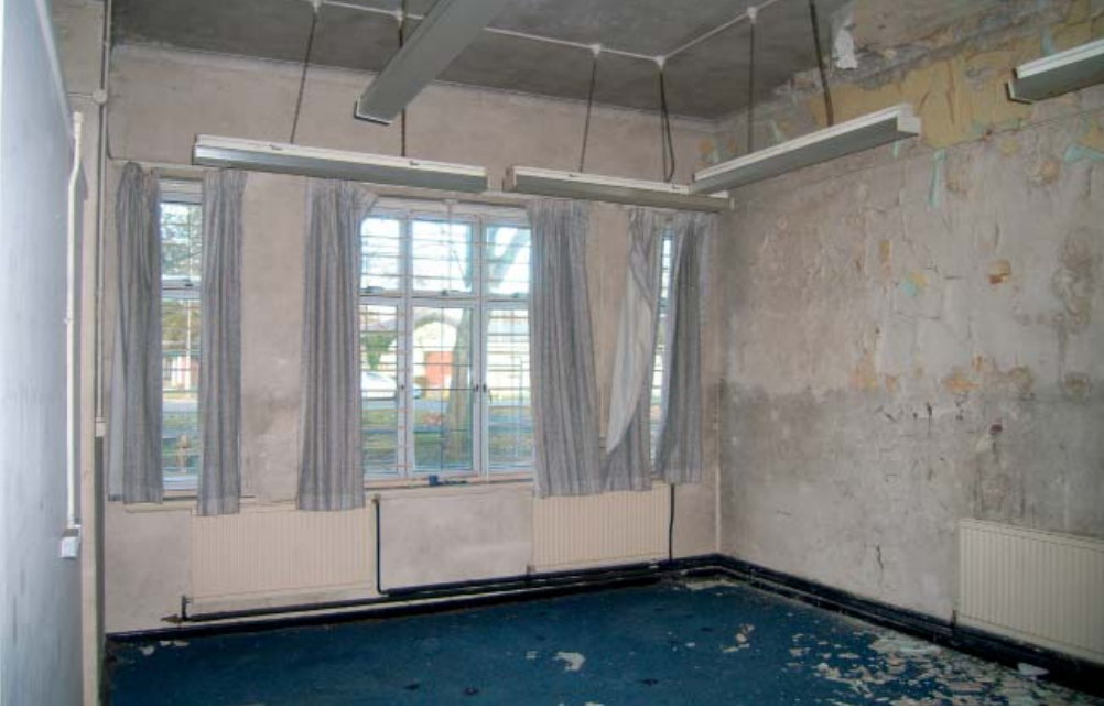
Plate 5: Ground floor room in main range of Building 455
