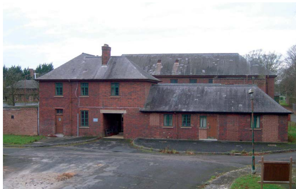
Plate 4: East side of Building 455
