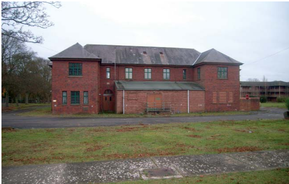
Plate 1: West front of Institute (B455) with extension to centre
