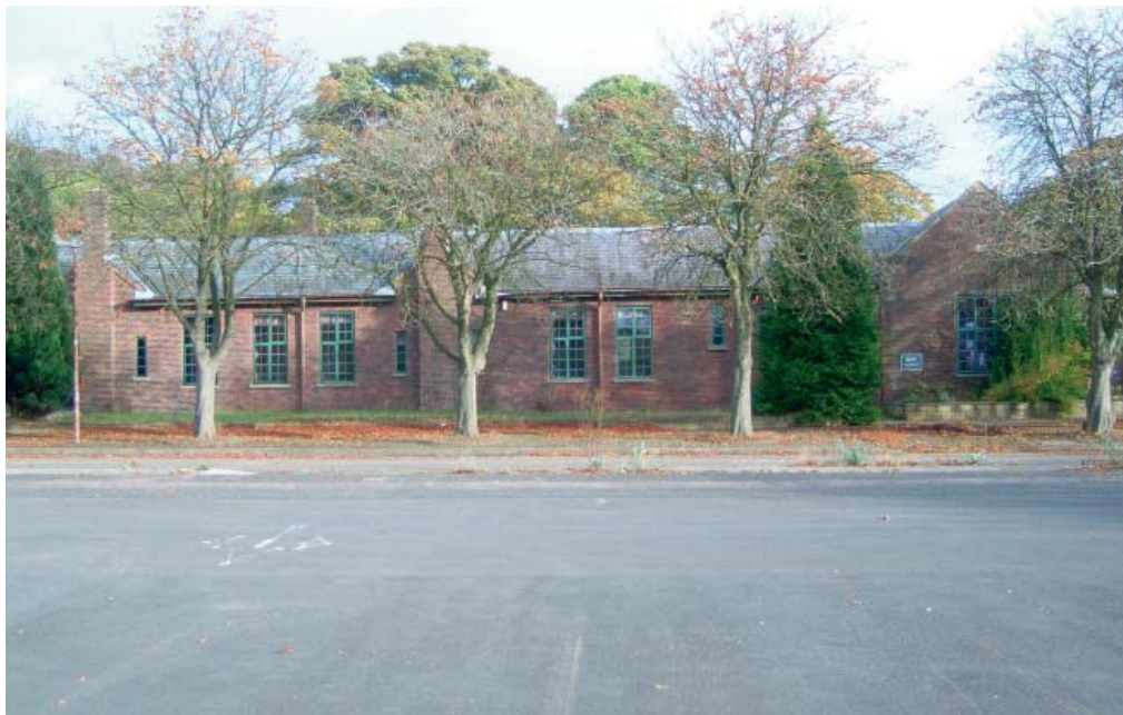
Plate 9: South elevation of Sergeants' Mess (Building 457)
