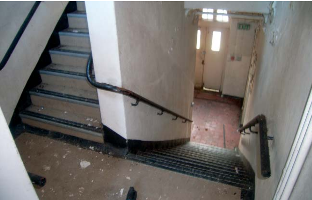
Plate 7: Staircase in Building 455
