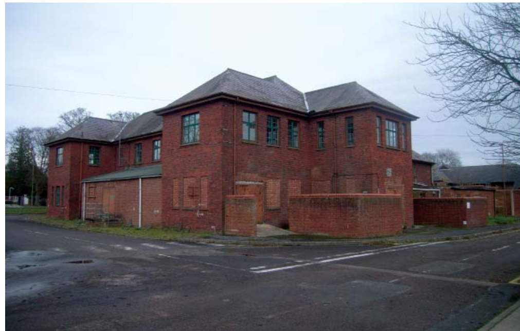
Plate 2: Building 455 from south-west
