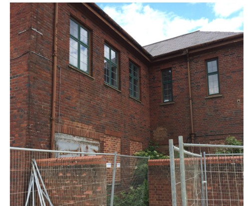
Demolition of courtyard walls
