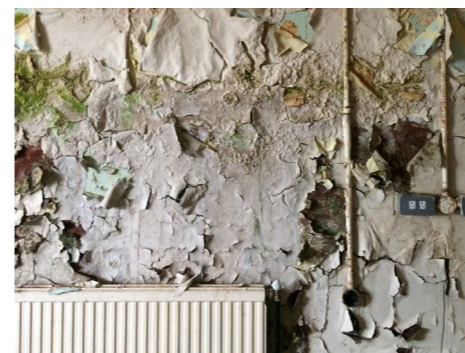
Damp brickwork
