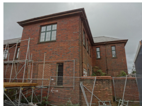
Re-instating bricked up windows
