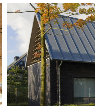
Metal standing seam roof finish
