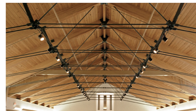
Glulam timber with slender steel bracing
