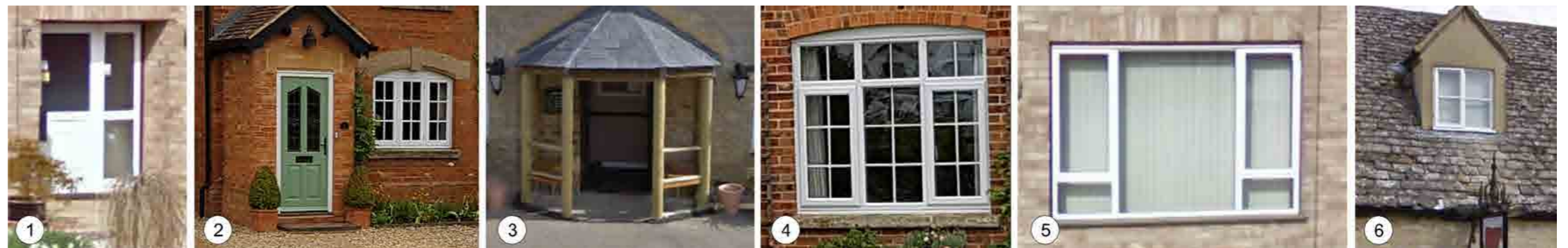
Window / Porch Details
