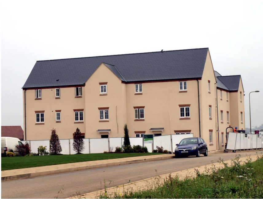
DEVELOPMENT EAST OF THE PARCEL ON THE AVENUE
