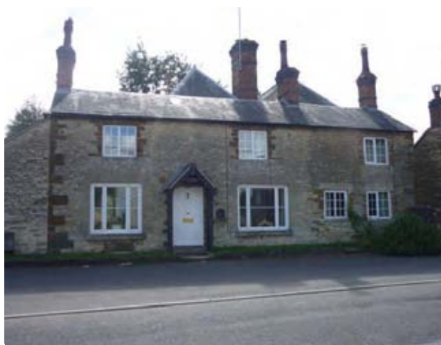
11. Chimneys can completely change the character of a building and should be retained on older buildings
