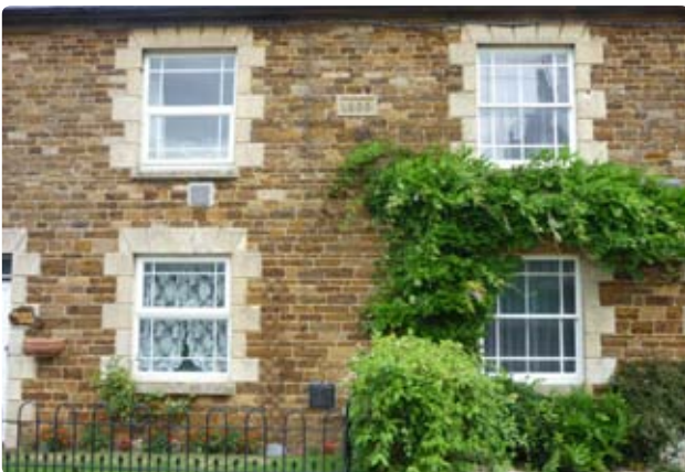
21. The heavier plastic windows to the left contrast with the slimmer and traditional timber sashes on the right
