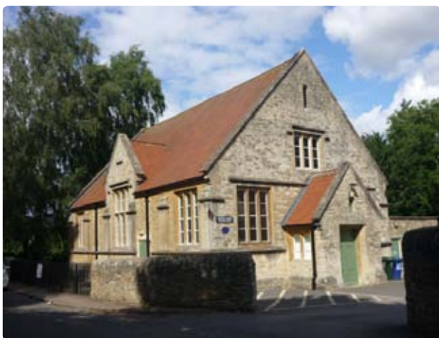
28. Village Hall, Fir Lane
