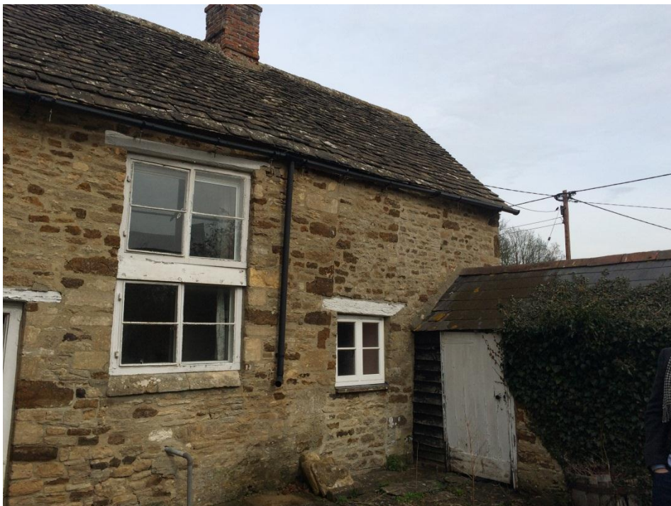
Photo 6 – View of rear projection and outbuilding
