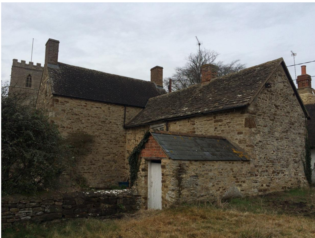
Photo 4 – rear elevation from east
