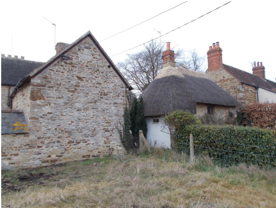
Photo 7 – from east to rear
