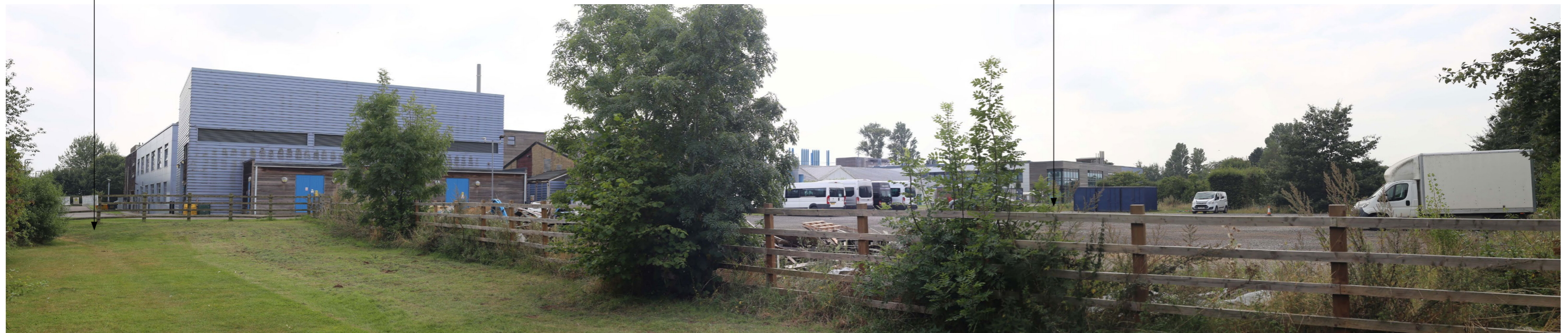
PHOTO VIEWPOINT Ib: View southwest from public footpath north of the IAT building (Institute of Advanced Technology)
