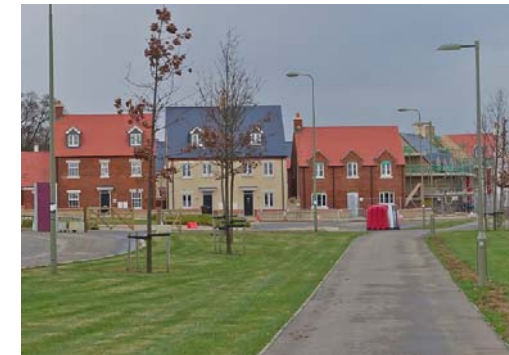
New residential buildings to road frontages
