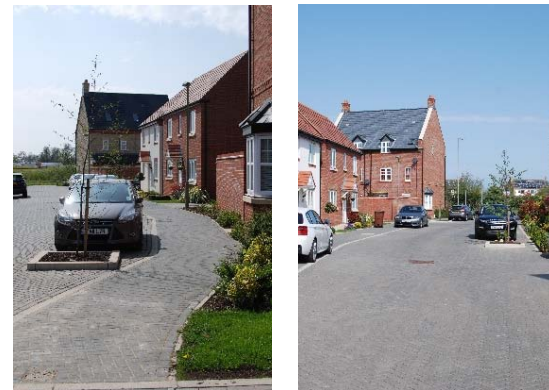
Views of present site and newly built access roads
