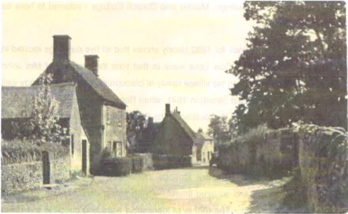
Early C20th photograph showing Chancel Cottage, with a large detached outbuilding in front of it.
