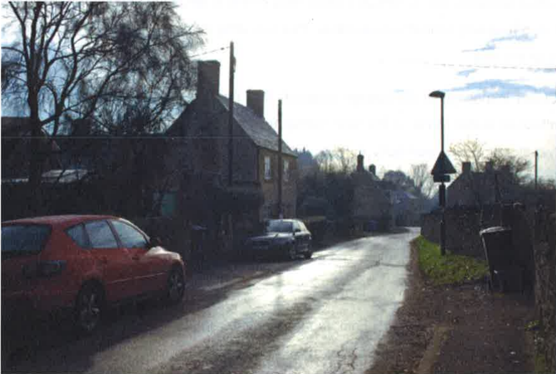
Note the difference in eaves detail from the photo above and also the loss of the outbuilding replaced with a flat roofed garage.
