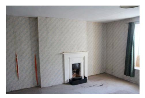
The floor is boarded with a fitted carpet, which is in poor condition. The floor boarding has been lined with hardboard, generally this appears to be in fair structural condition, but affected by condensation.
