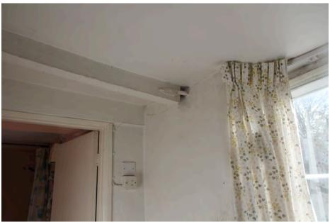
Photo showing the beam to the kitchen ceiling affected by the wall leaning outward
