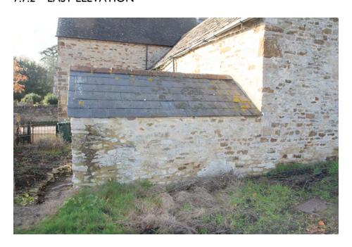
The east wall above ground acts as a retaining wall. There are slight movement joints to this to the corner to the south, general repointing is required. There is no gutter fitted to this outbuilding and this is recommended. The roof is slate with clay bonnet tiles, which is in fair condition.
