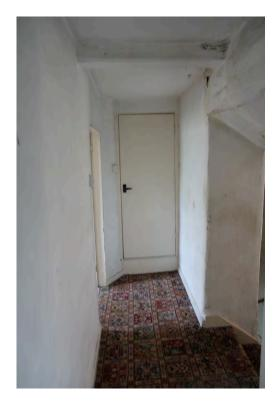
The floor is boarded with a fitted carpet, which is sound structurally. The walls are plastered.
