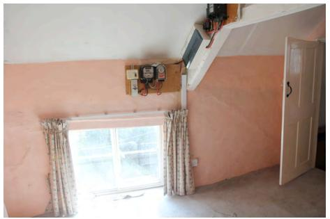
Photo showing the electrical incoming mains and distribution boards
