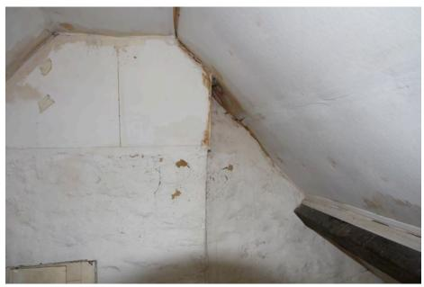
Photo showing the damage ingress to the north gable
