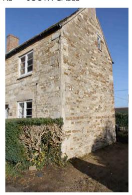
The south gable to the main range is in limestone rubble and ironstone, there are open joints to the corner to the west and at ground level, which require urgent repointing. The wall itself has been pointed in a hard cement mortar and some decay, consideration should be made to the replacing of this.
