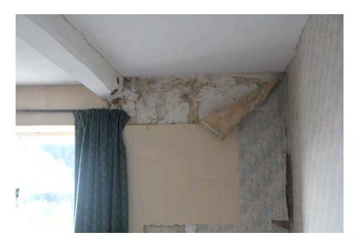
There is a cross beam spanning from east to west, which is in fair condition, the ceiling in lath, and plaster that has been lined with plasterboard and skimmed. It is unclear as to the condition of the lathe and plaster beneath this. There is some movement to the west wall where there is cracking to the plaster over the window, due to the wall moving outwards caused by the outward thrust of tying in of this is required.
