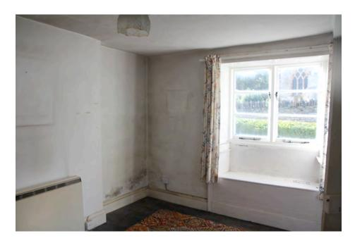
The floor is boarded which has been stained around the perimeter. The boarding generally is in fair condition. There are slight undulations to this. The walls have a moulded timber skirting fitted.
