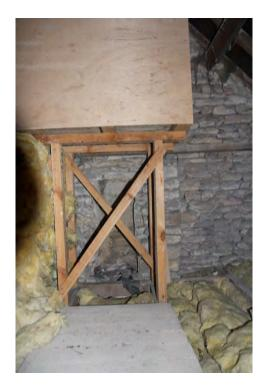
The ceiling joists to bathroom to WC have been replaced beneath the original timber beams, which span east to west, with a glass fibre quilt, which is disturbed and requires replacement. The walls are stone. To the west wall there is the gable wall, which contains the chimney breast. There is damp ingress from around the chimney. There are further movement cracks beneath the purlin. The water ingressing at the ridge has affected the end rafter to the roof where the ridge has rotted away.
