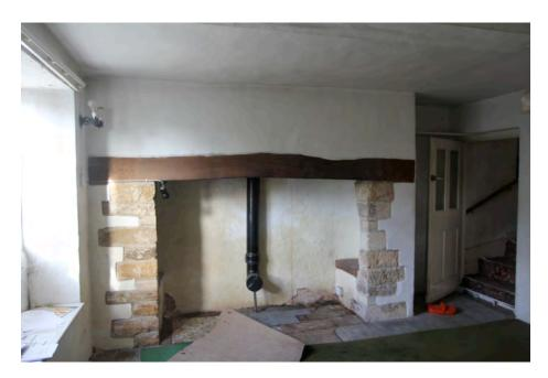
The floor is stone flagged which has been overlaid with hardboard and carpet, the stone flagging appears to be generally in reasonable condition except where it extends into the fireplace now removed was fitted. Here the floor is affected by damp to the centre of the area where there was a wood burning stove. The floor and the fireplace which has been reformed but replacement of the brickwork to the fireplace is recommended together with repointing.
