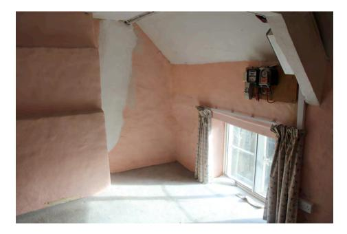
The floor is boarded with a fitted carpet. The floor has been lined with hardboard. There is considerable sag to the floor where settlement has occurred to the corner to the south east. The settlement to the extension is evident where the door has deflected and a make-up piece added.
