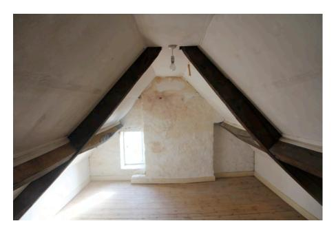
The Bedroom is formed into the roof space, which includes two trusses, with a central purlin to each slope. To the gable to the south there is a small single light window. The roof is formed into the roof space, which is lined with insulation board, this is taped to the joints and peeling and generally sagging, the upgrading of this is necessary. There is a small section of flat ceiling to the ridge. Water is ingressing to the centre of the roof.
