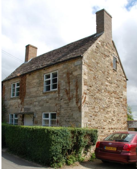
Chancel Cottage, from the SW.
