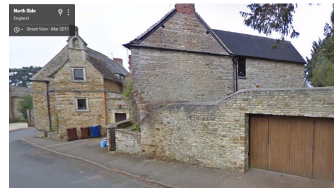
VIEW OF EAST ELEVATION OF EXTENSION FROM THE ROAD
