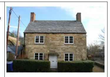
North Elevation Showing the extended rear elevation, the vertical joint in the stonework marking the later addition
