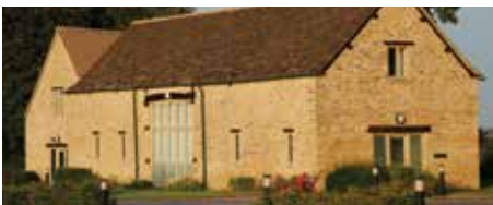
Barn Conversion Wing, England
