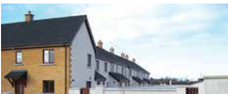
Social Housing Installation Co. Louth, Ireland
