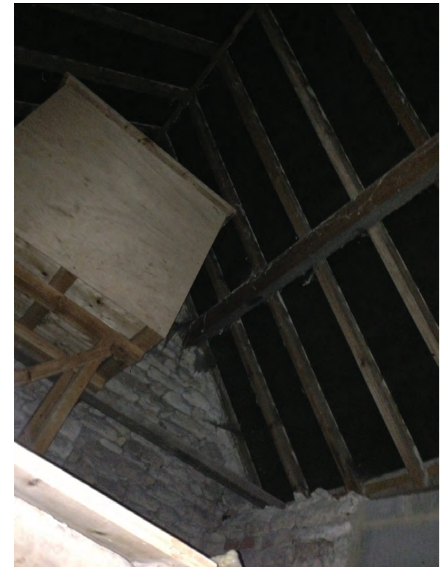
Fig.28 - Bathroom roof space
