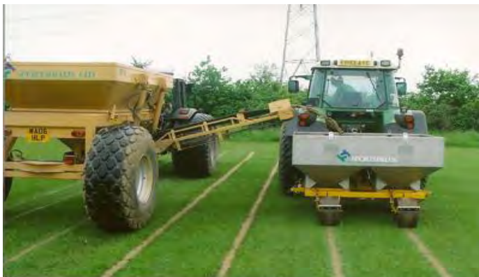
Installation of Secondary Slit System
