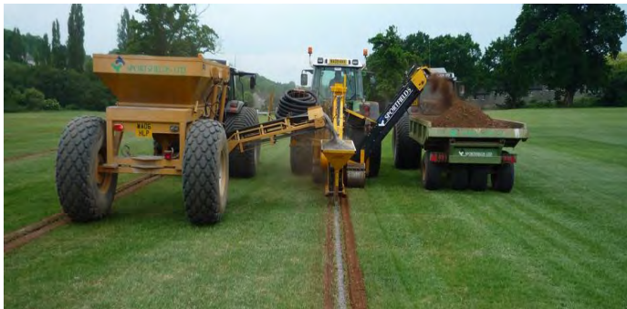
Installation of Primary Piped System
