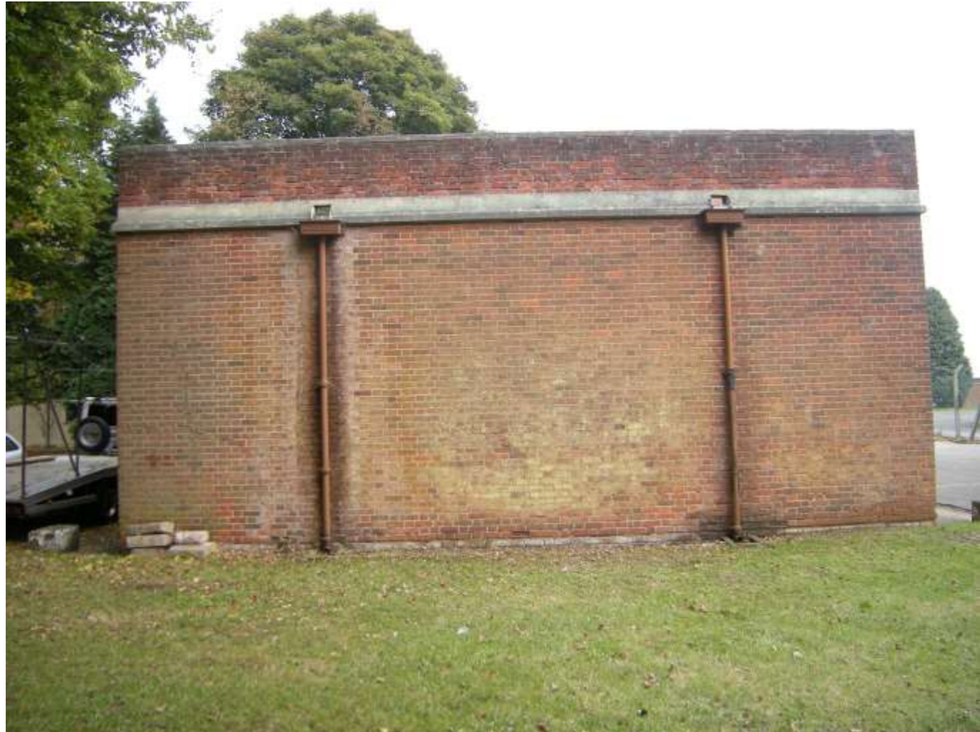
Building 105-view from south west
