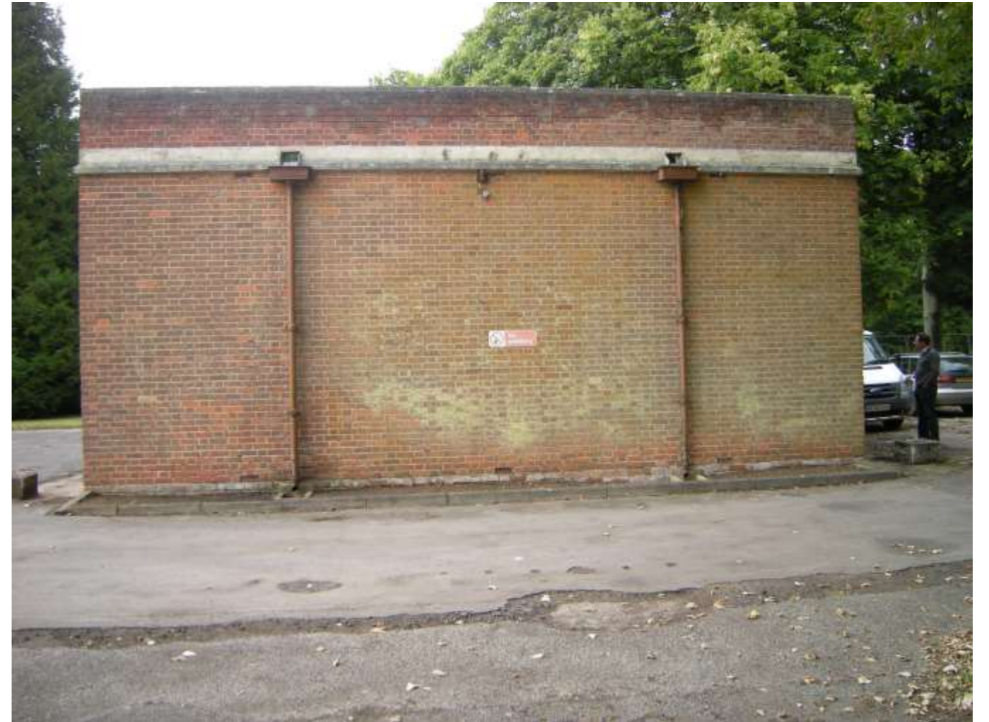
Building 105-view from north east
