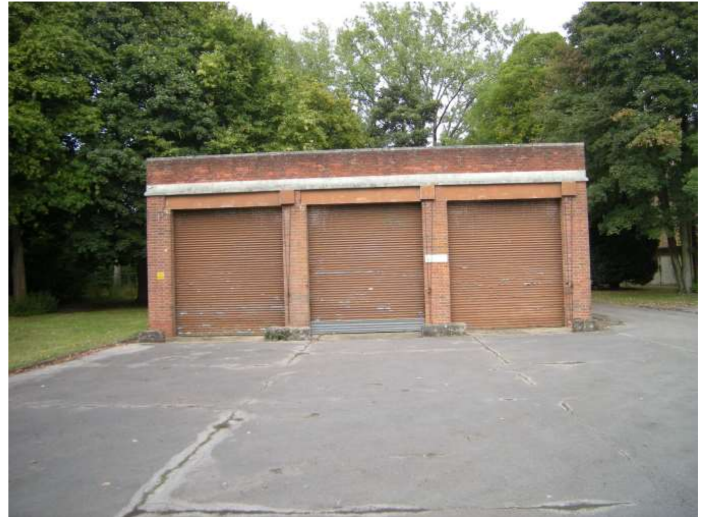
Building 105-view from south east
