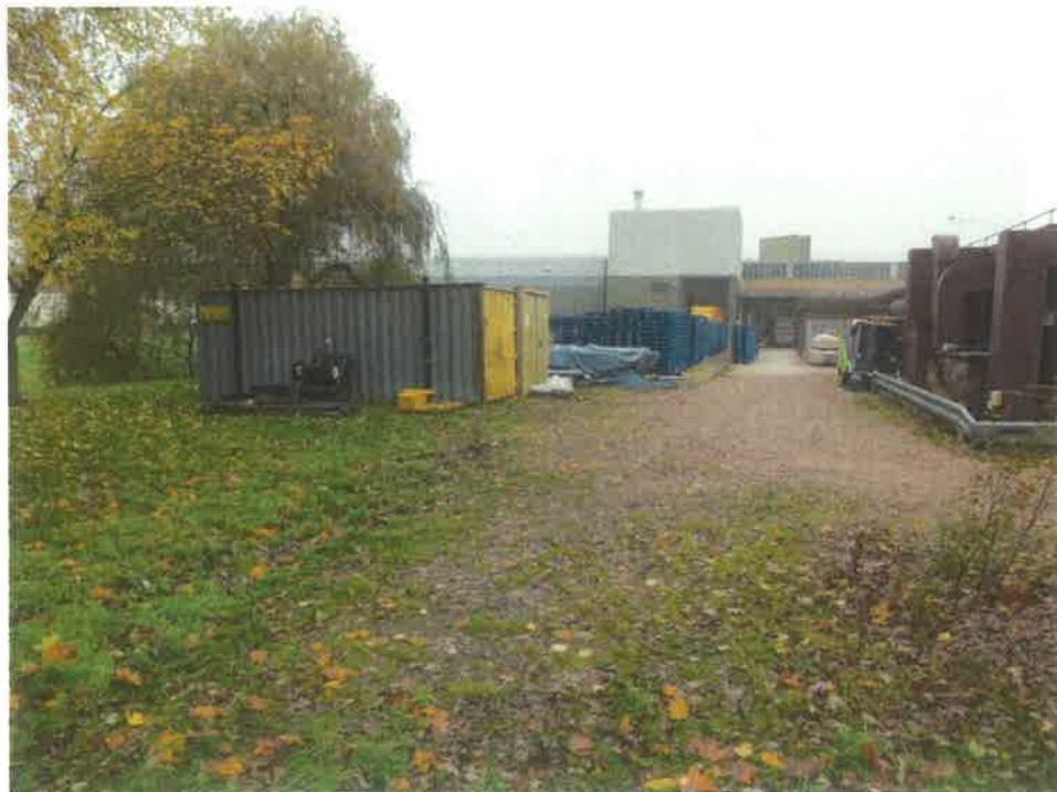
Photo 12: View of pallet storage area located in the north-west corner of the site, looking west.
