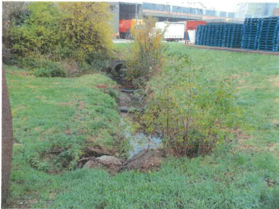
Photo 6: View of Birds Brook as it emerges from a culvert looking west. There are two booms across the brook channel at this location, presumably to contain any accident discharges of pollution to the watercourse.
