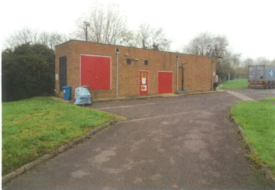
Photo 3: View of electrical sub-station located beyond the south west corner of the study site boundary, looking south west from the southern site boundary.
