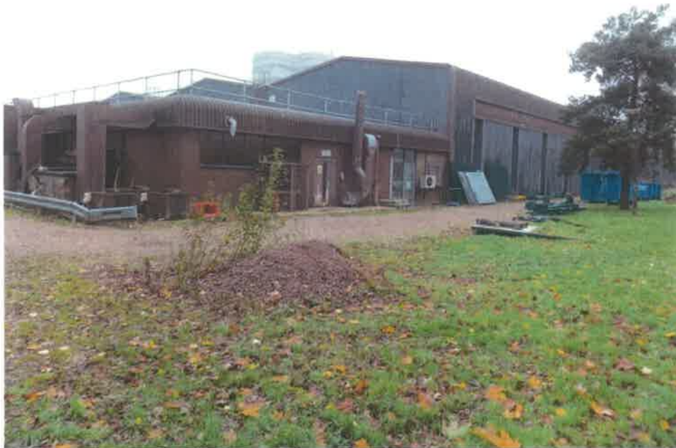
Photo 11: View towards factory building located beyond the northern site boundary, looking north-west. This building is labelled as "Max Pax Building" on the Kraft topographical survey.
