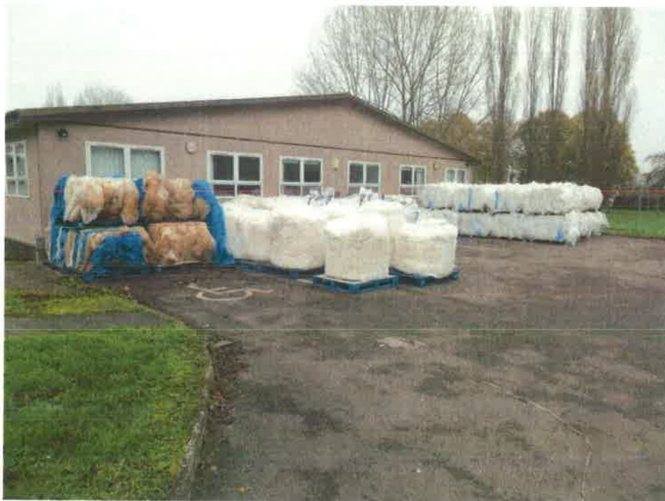
Photo 2: View of southern end of vacant office building and car park looking north-east from southern site boundary. The materials on the pallets were packaged and bound, probably awaiting off-site recycling.
