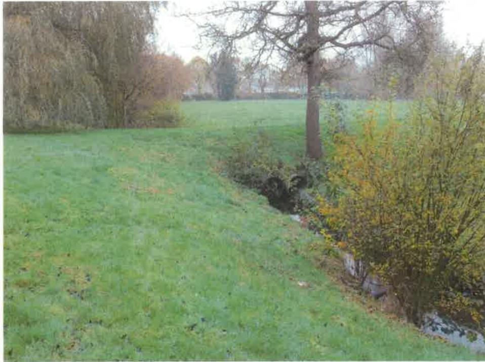
Photo 7: View towards earth "bridge" over Birds Brook in the north-western corner of the study site. The watercourse flows through two circular concrete pipes over this short section.
