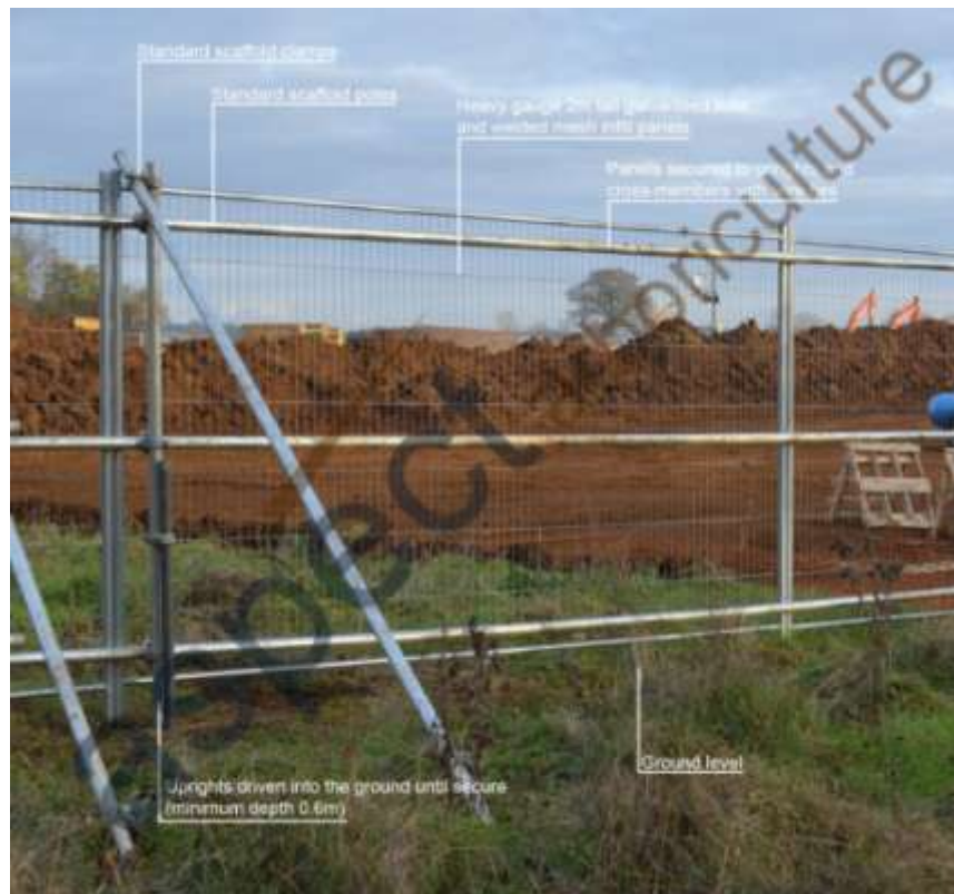
Plate.1 Default Protective Barrier Specification
