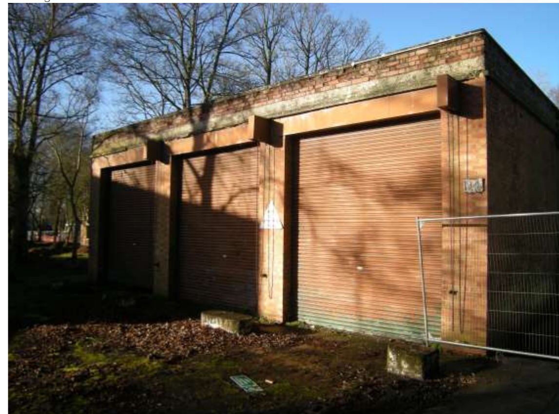
Building 94-close up view from south
