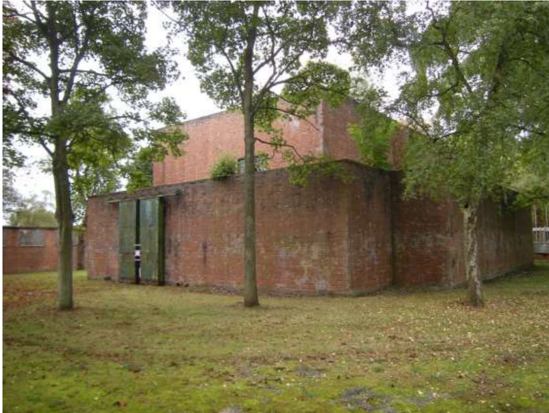
Building 93-view from west
