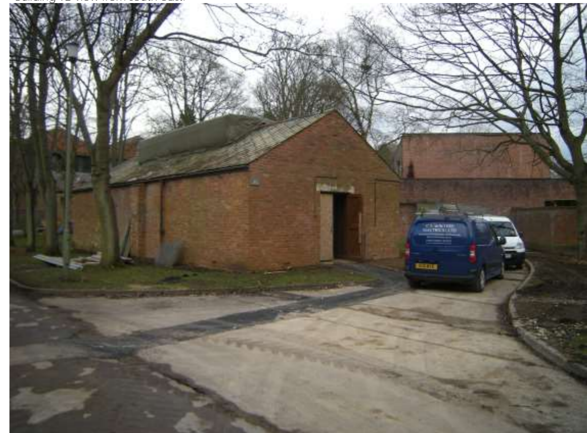
Building 92-view from north west
