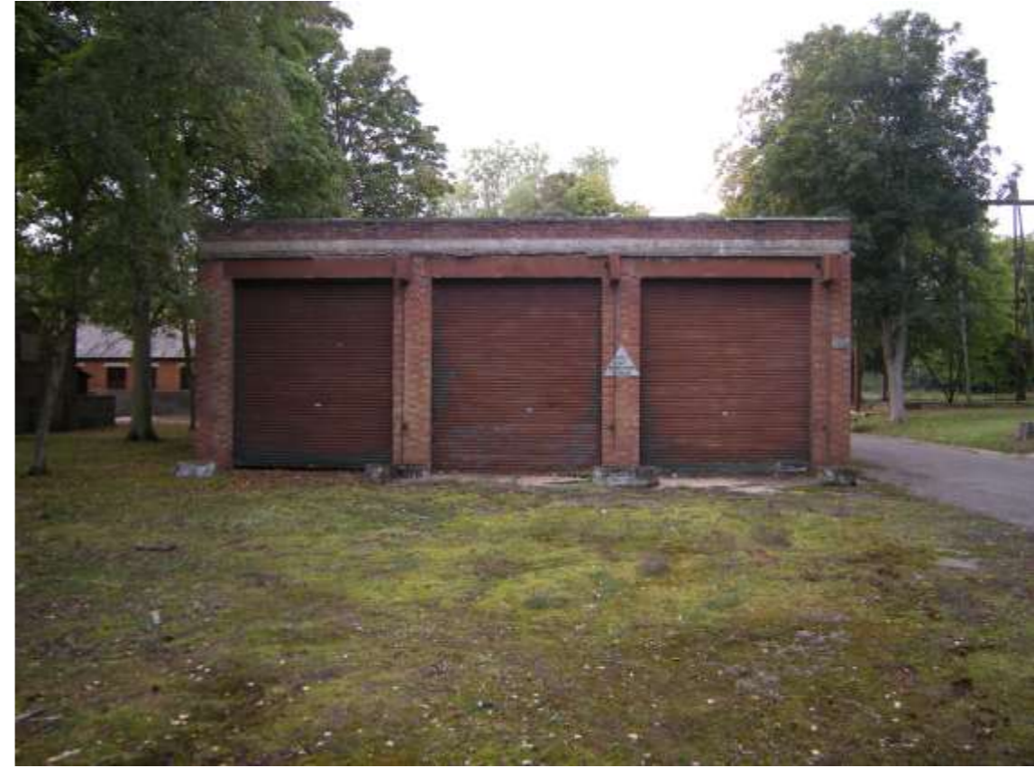
Building 94-view from south
