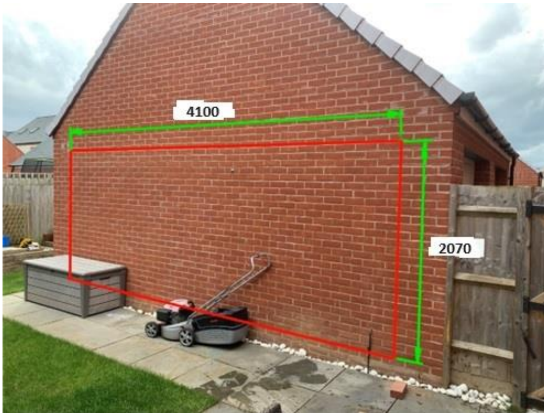
Image 4: Garage to garden wall cutout size for bi-folding doors in mm. (not to scale)
