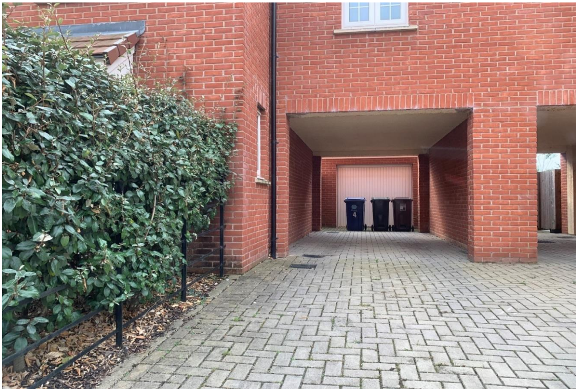
Image 3: Original car port and front parking space for 2 cars (see image 11)
