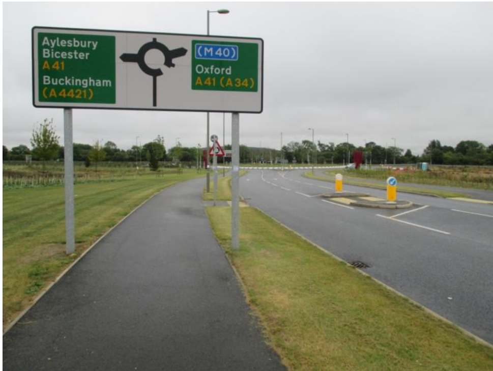
Figure 4. Vendee Drive Footway / Cycleway
