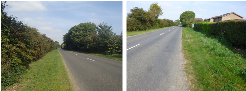
Lack of Pedestrian Facilities along Howes Lane (A4095)
