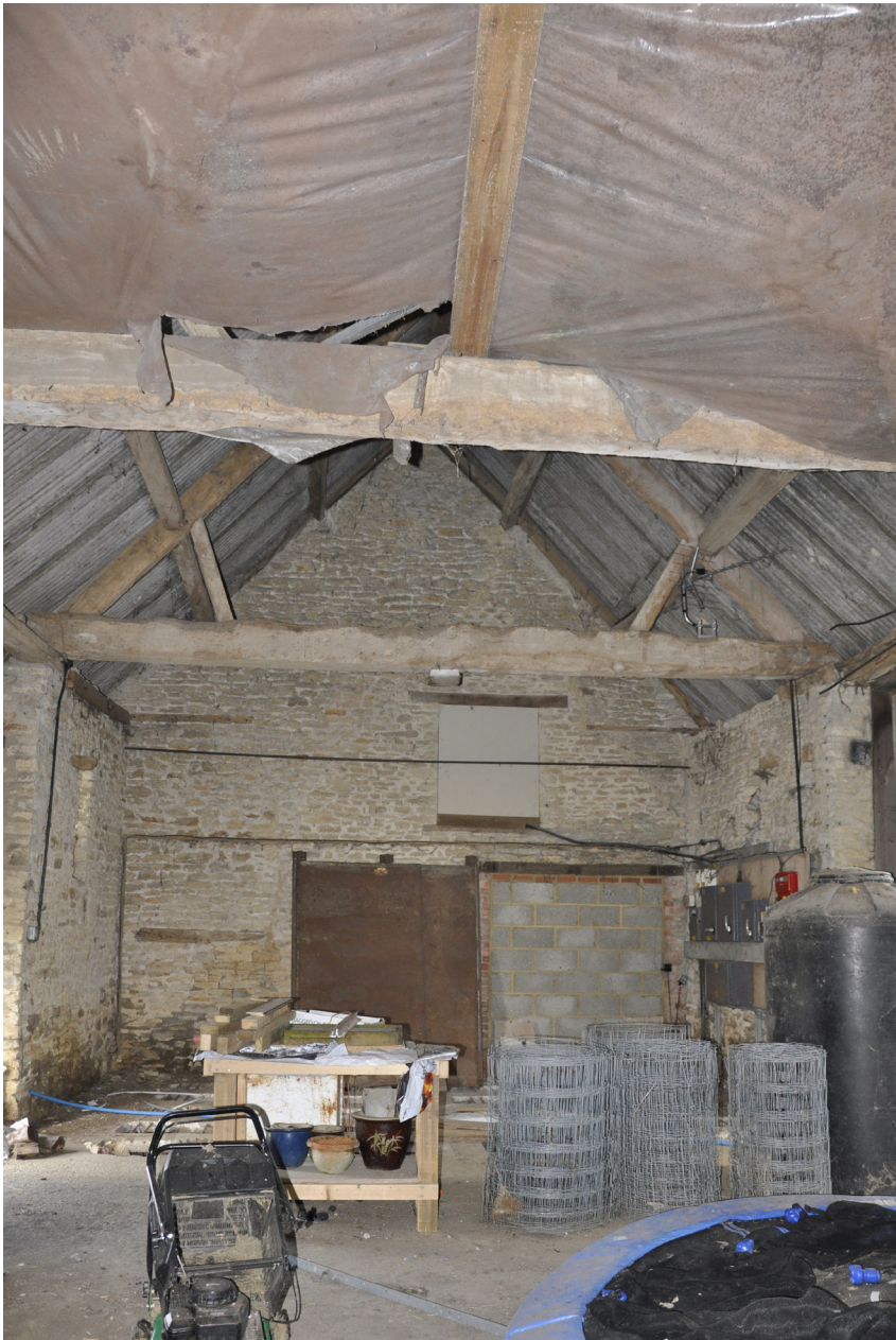
The roof structure of the southern barn, thought to be original
