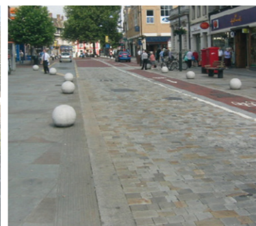
E5- Change of road surface material/ colour
