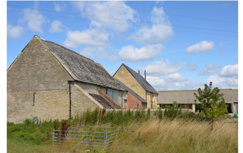
View from the south of the Grade II listed barns
