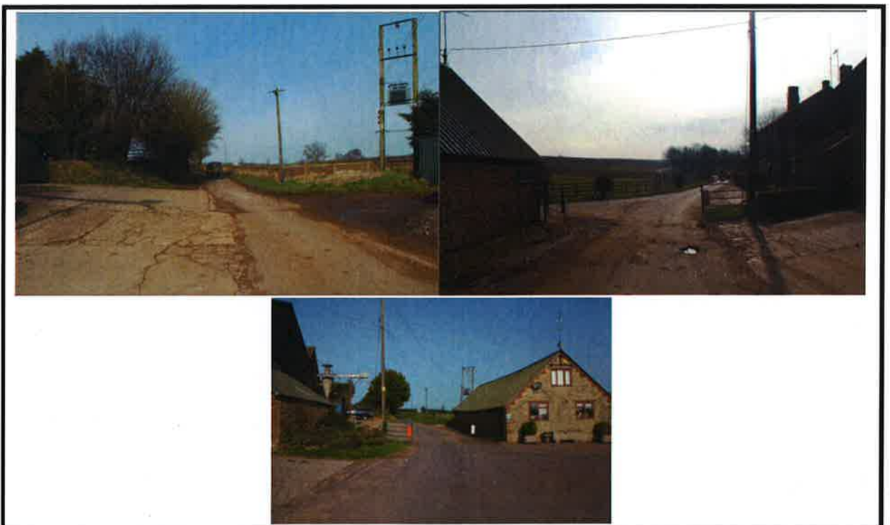
View to and from the junction with Park Lane.
