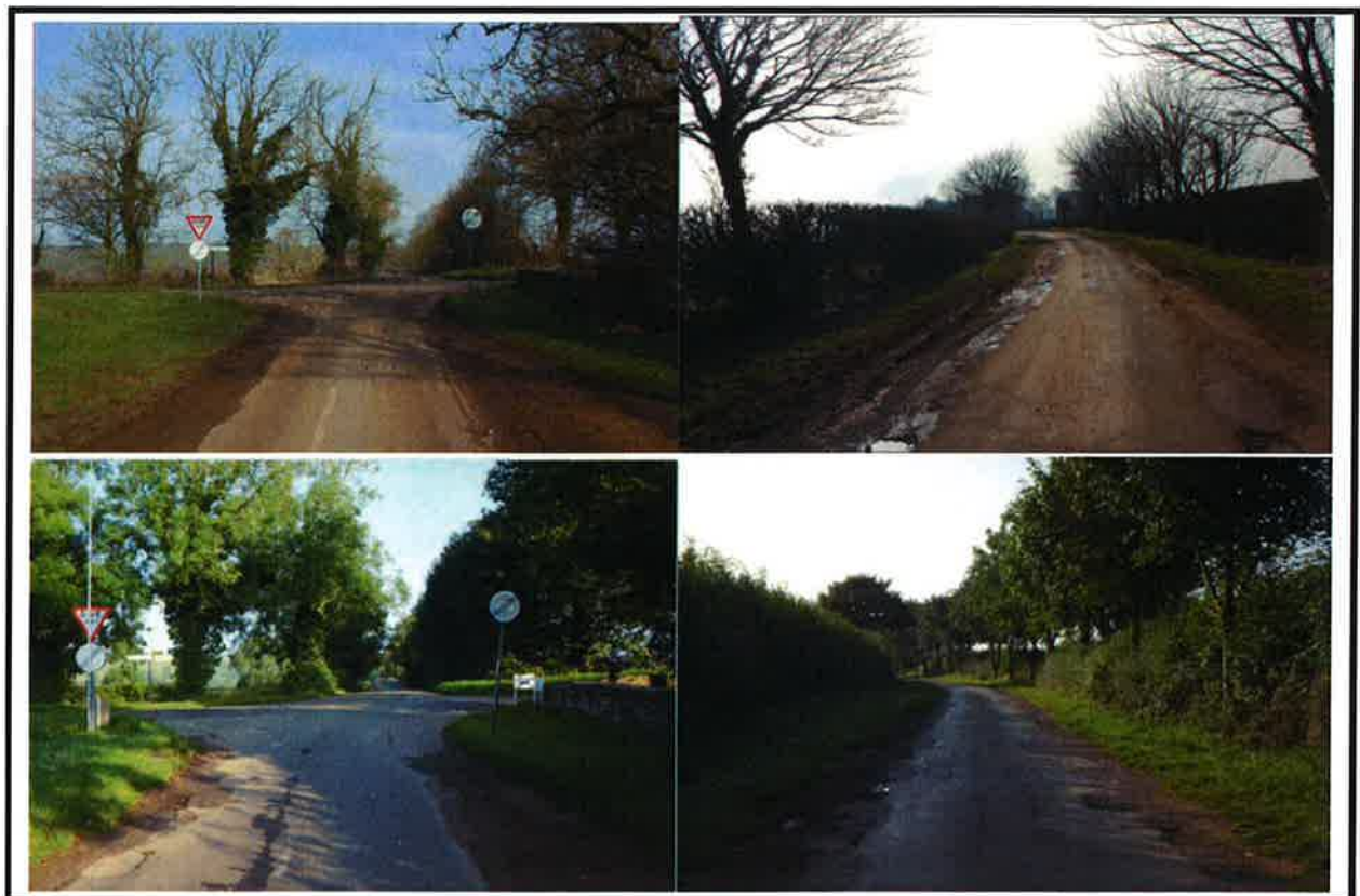
View to and from the junction with Main Street.
