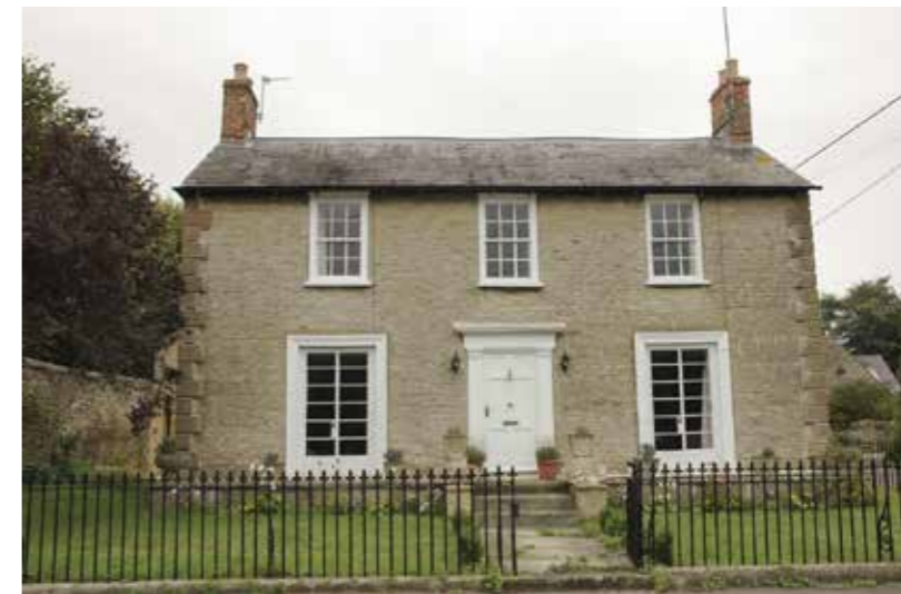
'Formal' stone building with symmetrical facade and dressed stone quoins.
