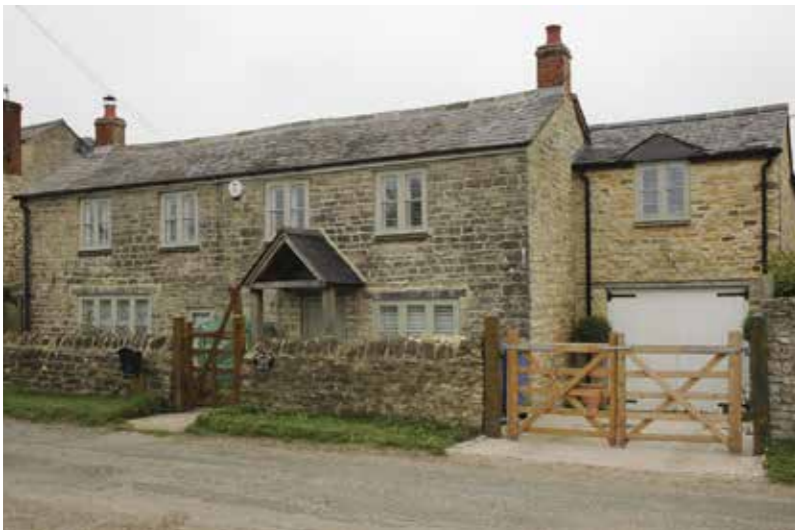
Timber details on boundary features.
