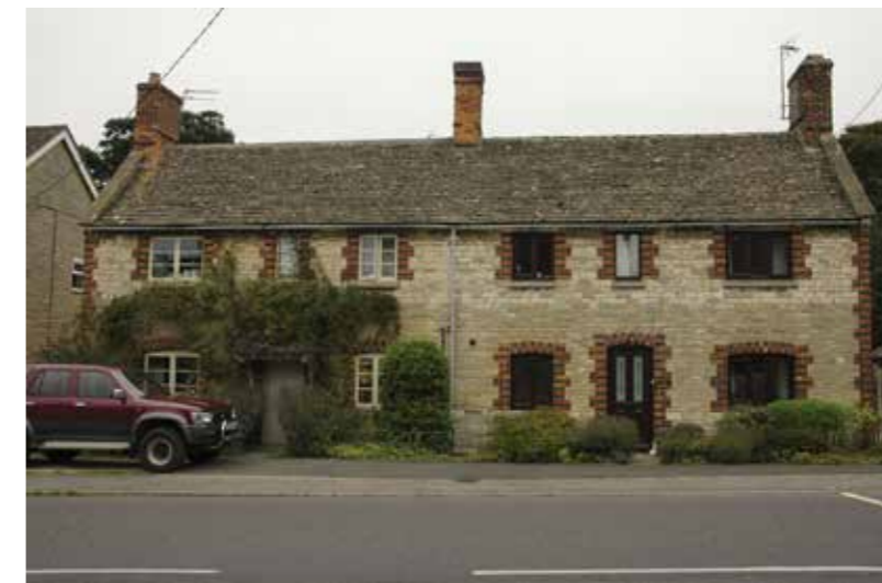
Pair of dwellings defining built in stone with red / blue brick details.
