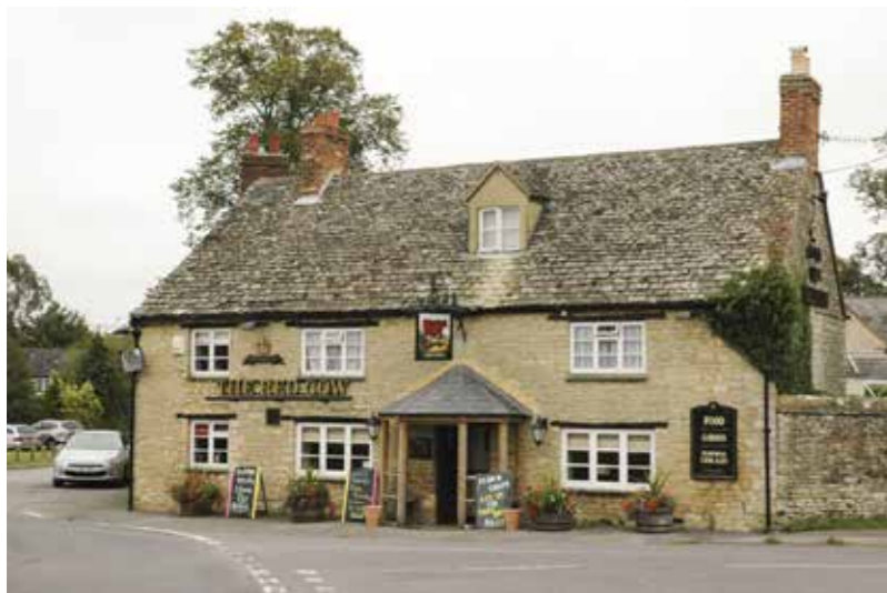
Simple stone building with pitched dormer and door canopy.
