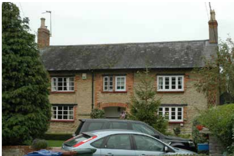
Stone as a main facing material with red brick details to windows and doors.
