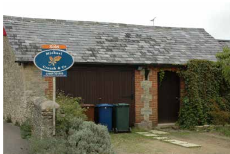
Stone with red brick details to garages.
