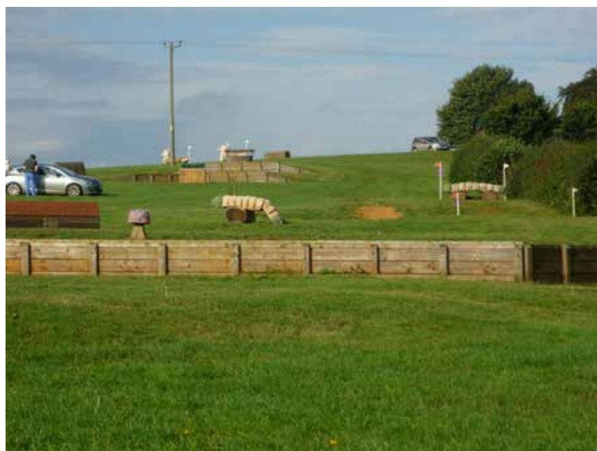
Permanent Fences constructed without Planning Permission
