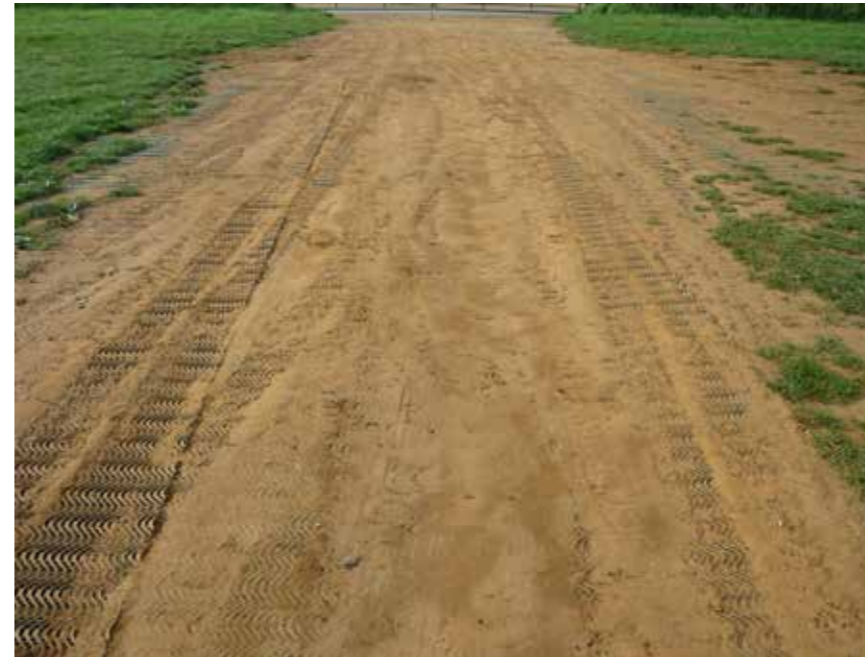
Grid at the Unauthorised Access from Main Street
