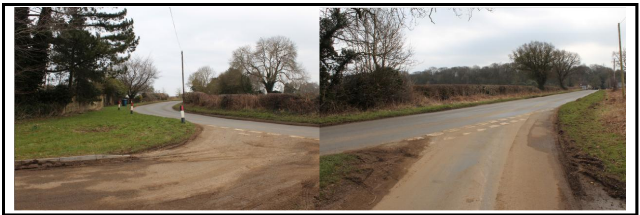
View left and right from Park Lane
