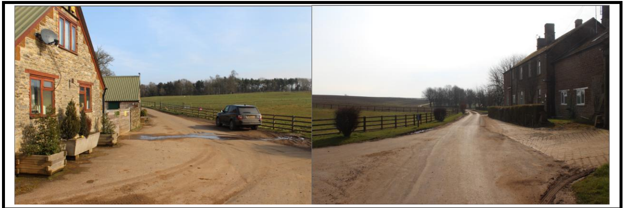
View left and right from junction with Park Lane.
