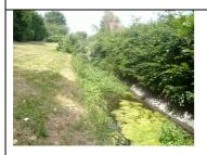
Immediate upstream of the culvert on Middleton Stoney Road, the Brook is lined having trapezoidal shape. The section is 1.2 m deep, bed is 2.0 m and side slope is 1:1.
