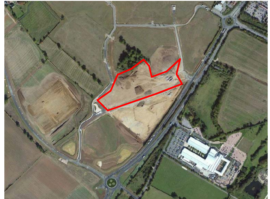
Fig.2 AERIAL VIEW OF PLOTS KM7 & KM9, KINGSMERE
