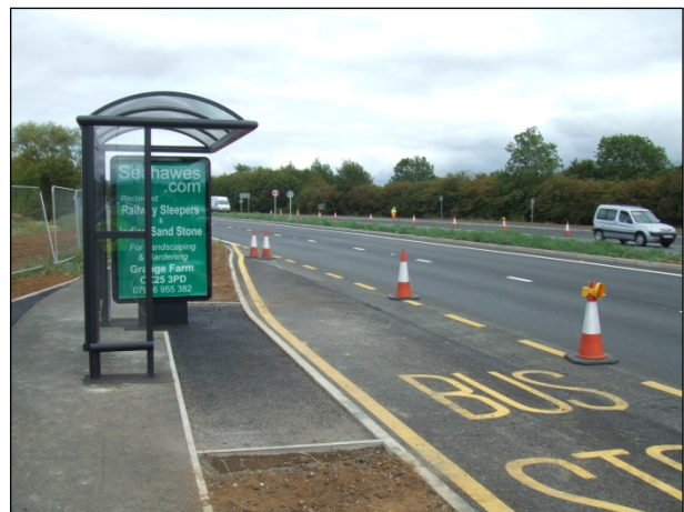
Photo 4 – Bus Stop and Footway Improvements Adjacent to the A41
