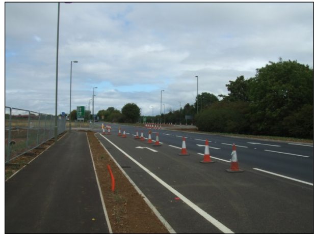
Photo 2 – A41 Looking North Towards Bicester and the New Junction
