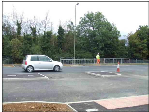
Photo 6 – Pedestrian Crossing Provision Over A41 Southbound Carriageway
