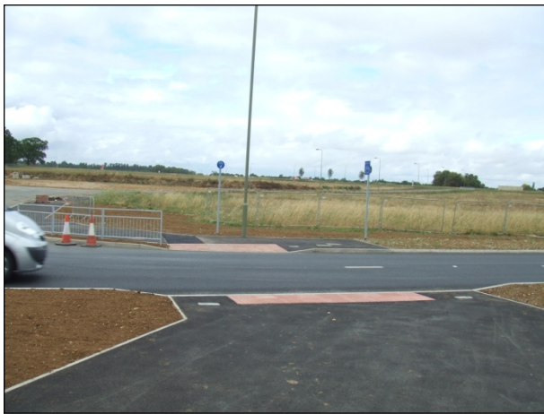
Photo 5 – Pedestrian Crossing towards the Premier Inn Site Over A41 Northbound Carriageway
