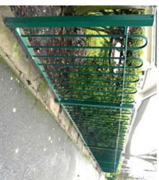
1.00m high box top fencing, colour black, with 1.20m wide self-closing gate.
