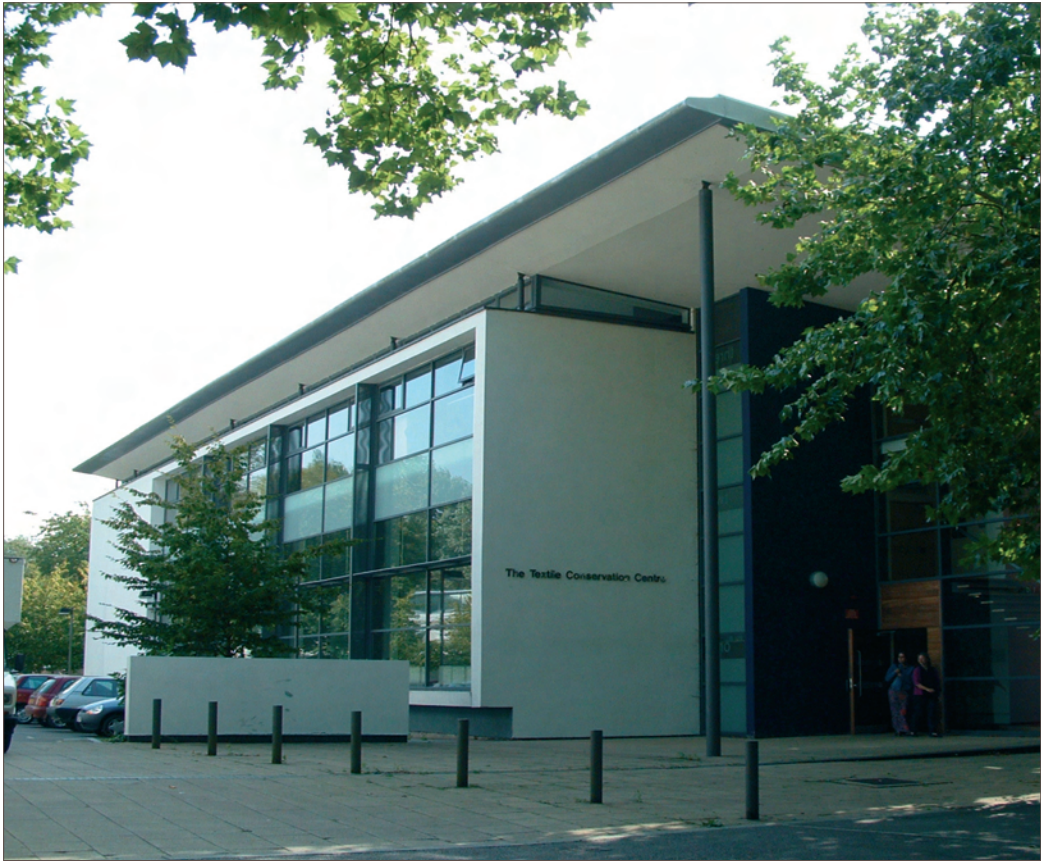
Public buildings and areas of civic significance in the Health Village must be of the highest quality, assessed in terms of functionality, innovation and robustness (in both the short and long term), as well as in the standard of materials and detailing used.
