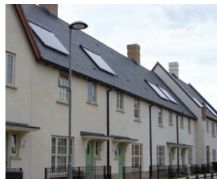
Roof-mounted solar heating panels (Upton, Northampton)
