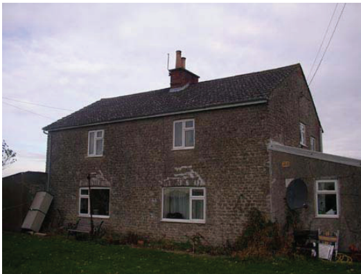
Figure 1 Southern and eastern elevation
