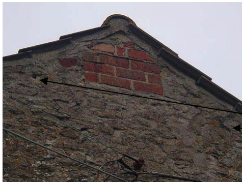
Figure 5 Holes in eastern elevation
