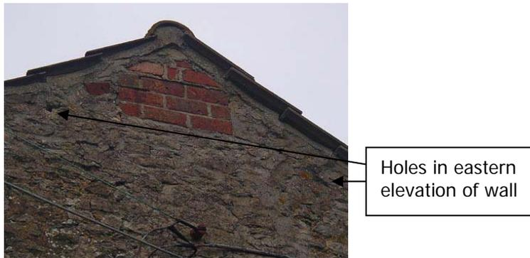
**Figure 5** Holes in eastern elevation
