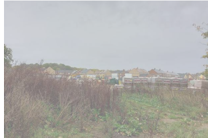
View of the adjacent residential development (Phase 1) under construction
